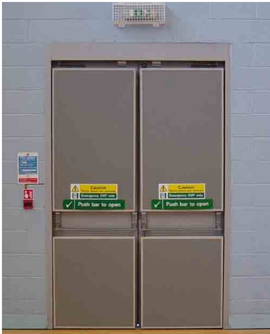
Sports hall walls should be detailed for safety and without hazardous projections. Flush surfaces should extend to 2.0 m minimum, preferably to 2.7 m above floor.
