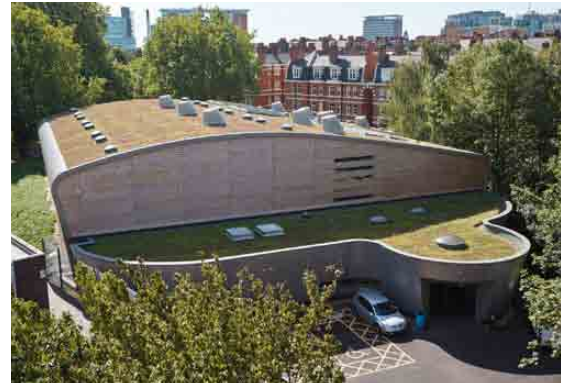
Natural ventilation towers in roof to give controlled ventilation and compensate for the heat loads from occupants, artificial lighting and solar gain, and anti-glare roof-lights to supplement the artificial lighting
