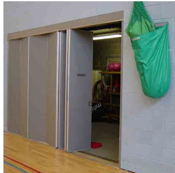
Store doors should be flush detailed, and unless they can only be opened by operators and otherwise kept locked, they should not open out into the sports hall. Doors may need to perform as rebound panels and therefore their construction needs to be robust and safe for users. Net bags should have no projecting fittings/features that could create a hazard and be high enough to not compromise the five-a-side rebound zone (1.21 m).
